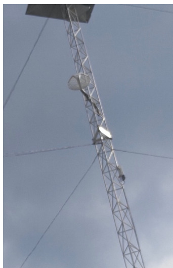
(b) Wireless router and wireless access point
